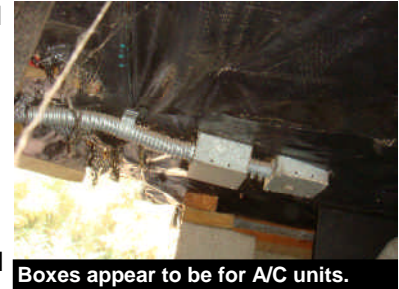
Boxes appear to be for A/C units.
