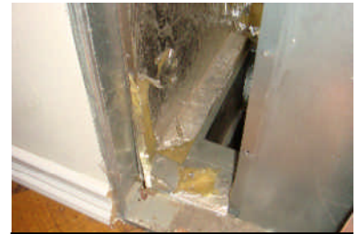
Damaged & soiled return & insulation.
