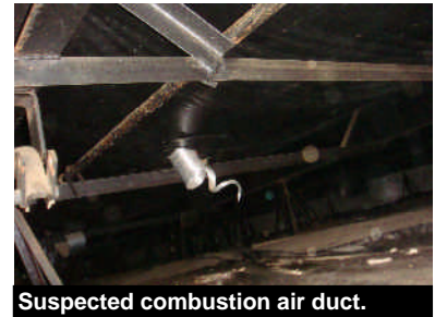
Suspected combustion air duct.
