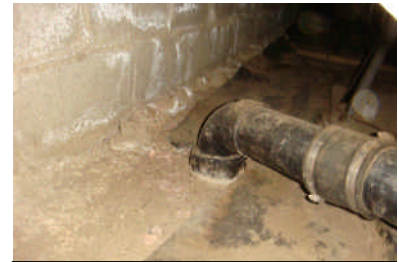
Main drain pipe termination location.
