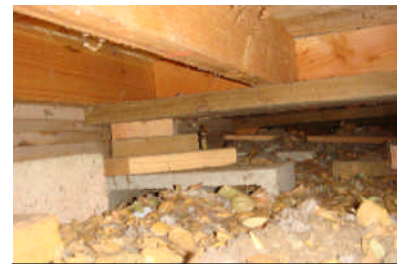
Improper office floor support.
