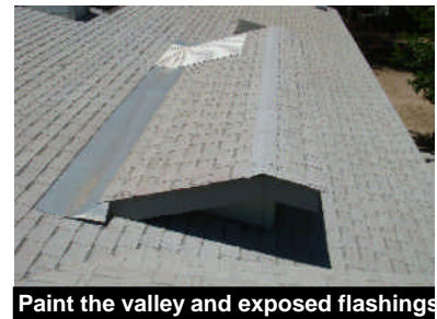
Paint the valley and exposed flashings
