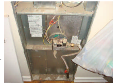
Damaged & soiled return & insulation.
