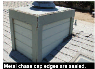
Metal chase cap edges are sealed.
