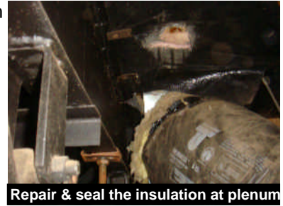
Repair & seal the insulation at plenum
