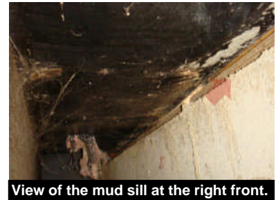
View of the mud sill at the right front.
