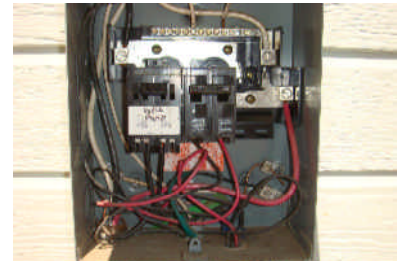
Panel at the right side of the building.
