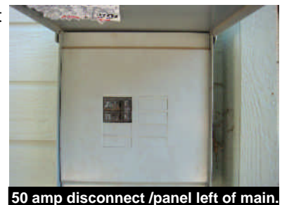
50 amp disconnect /panel left of main.
